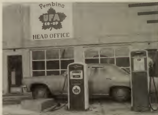
The Head Office of the Pembina U.F.A. Co-op Association.
